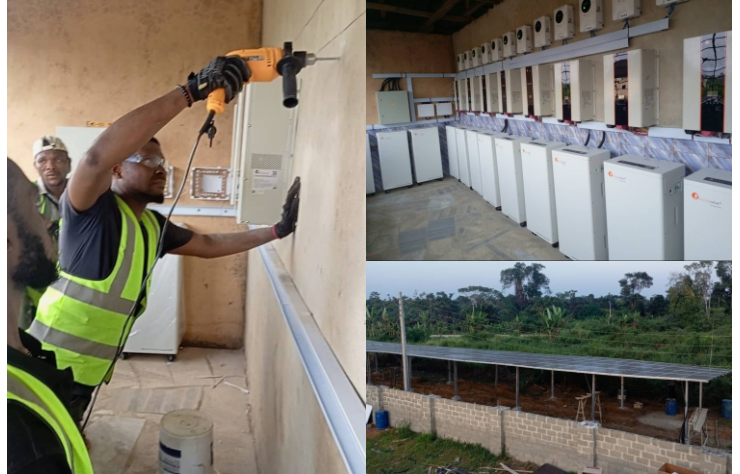
Installation of 80kva, 72KW(PV), 180KWh(BESS) at Okomo Community, Edo State, Nigeria
